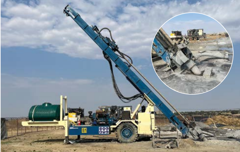
Regergen has drilled, designed and built the country's first commercial LNG plant.
