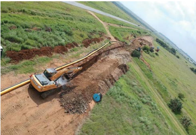
Pipeline being laid.
