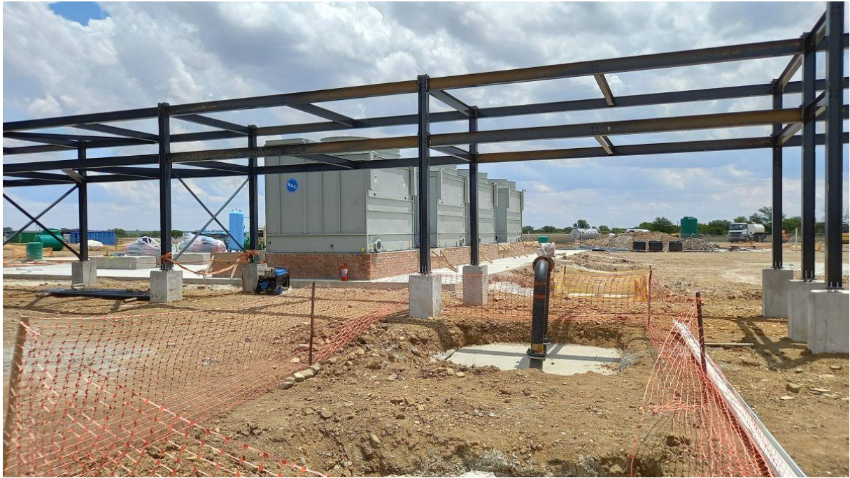
Figure 14: Installation of the fire water pipeline continued.
