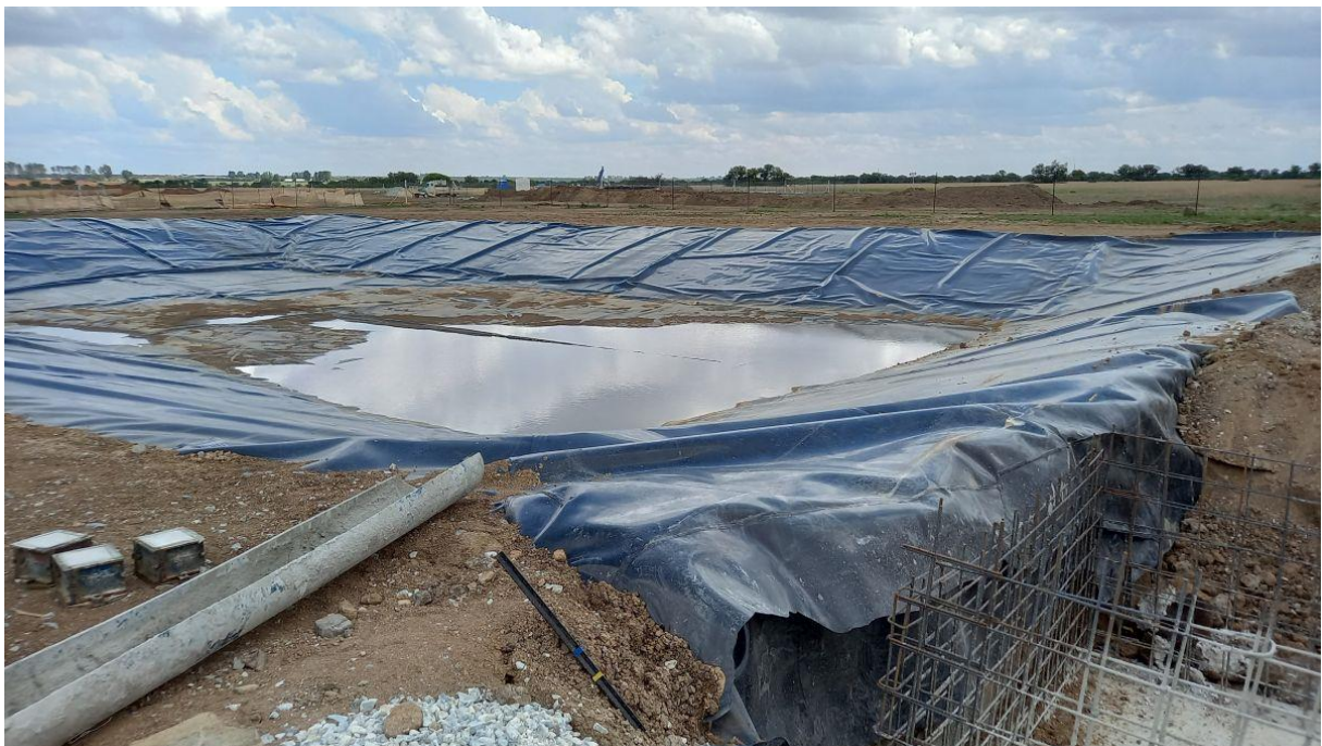
Figure 15: Construction of the PCD and associated infrastructure continued.
