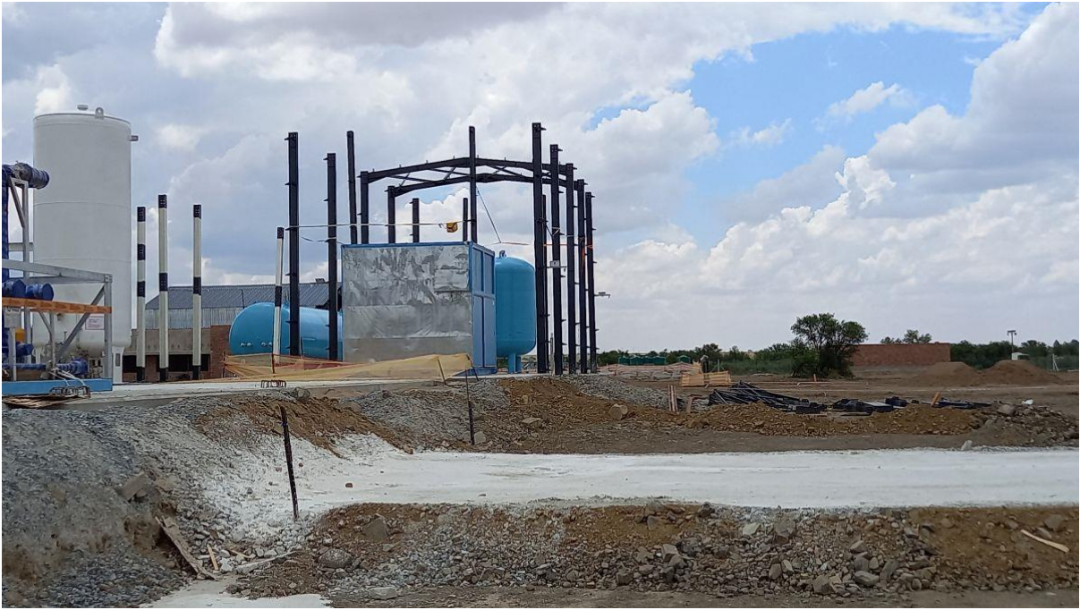
Figure 12: Installation of the canopy over the helium storage tanks continued.
