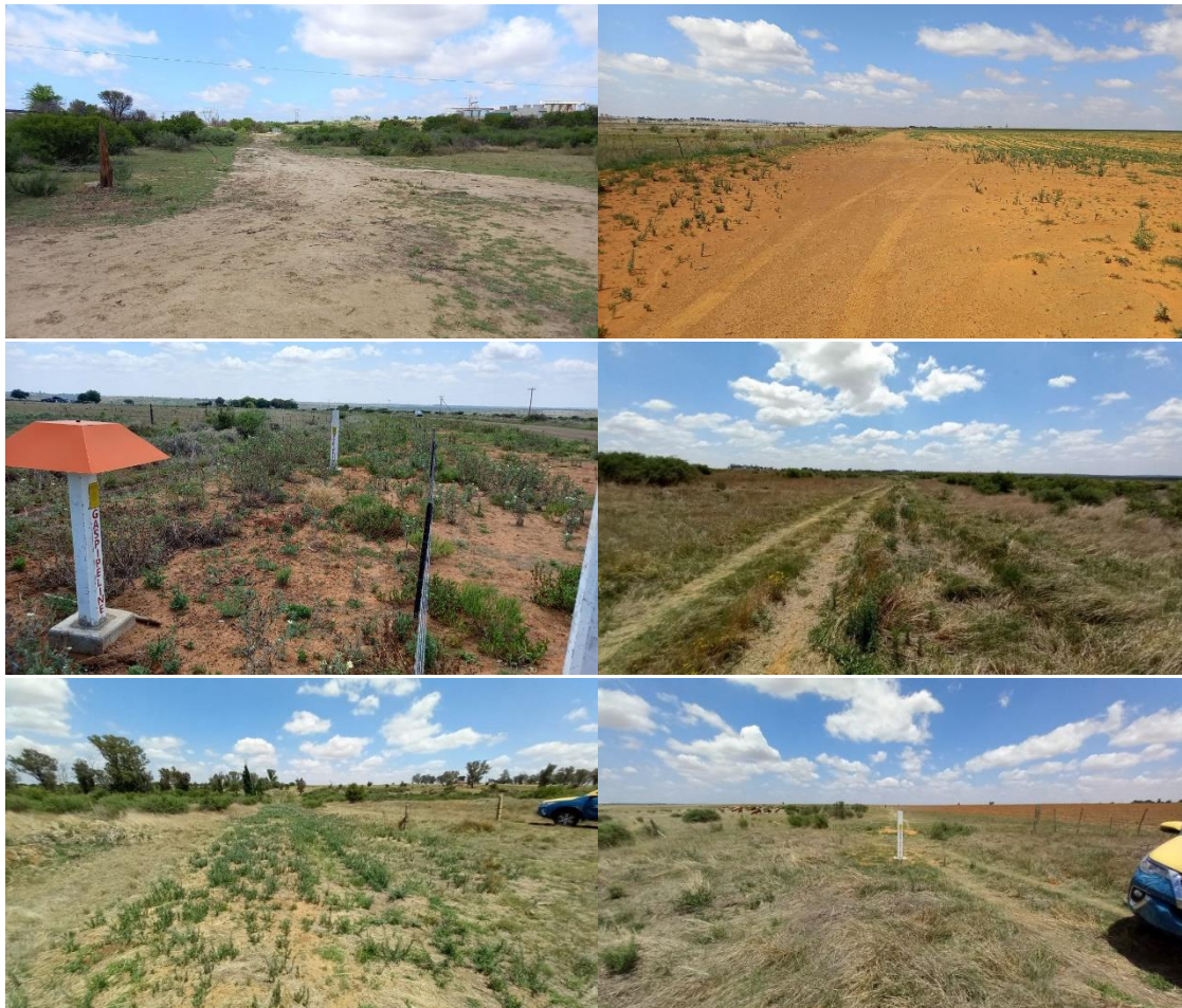
Figure 7: Rehabilitated areas along the pipeline route from well 2057 to Compressor Station A.
