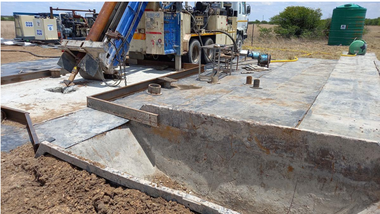
Figure 17: Site preparation for drilling of well P15 was completed.
