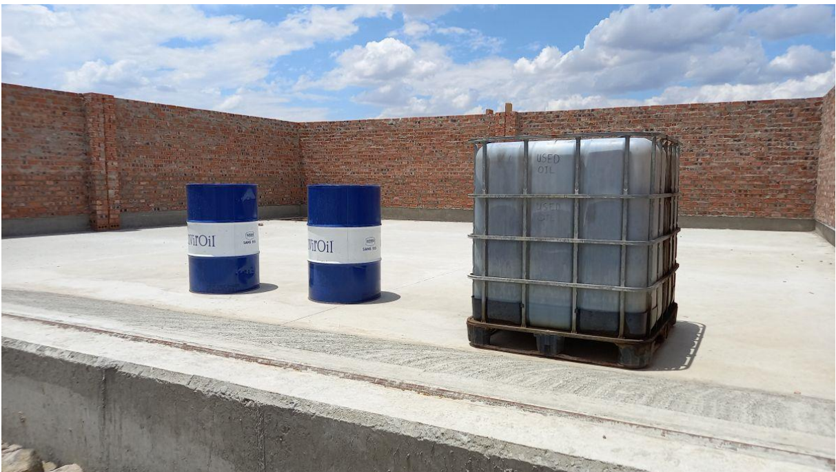
Figure 11: Construction of the operational waste storage area.
