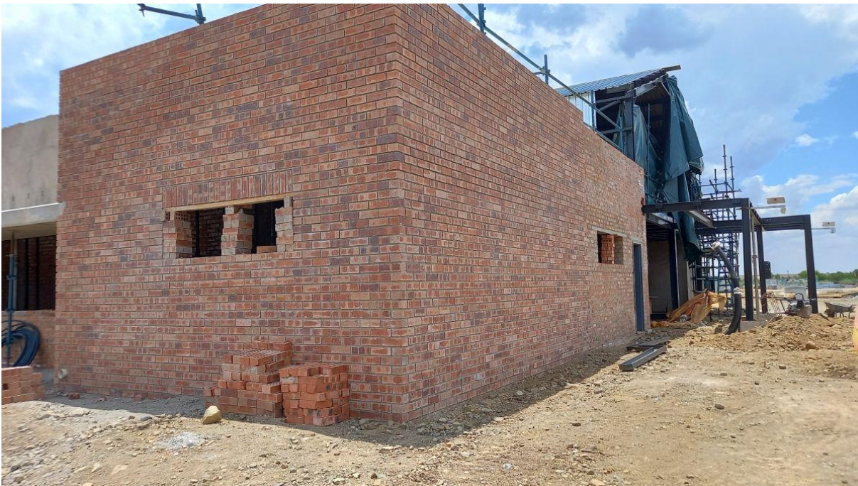
Figure 13: Construction of the MCC building continued.
