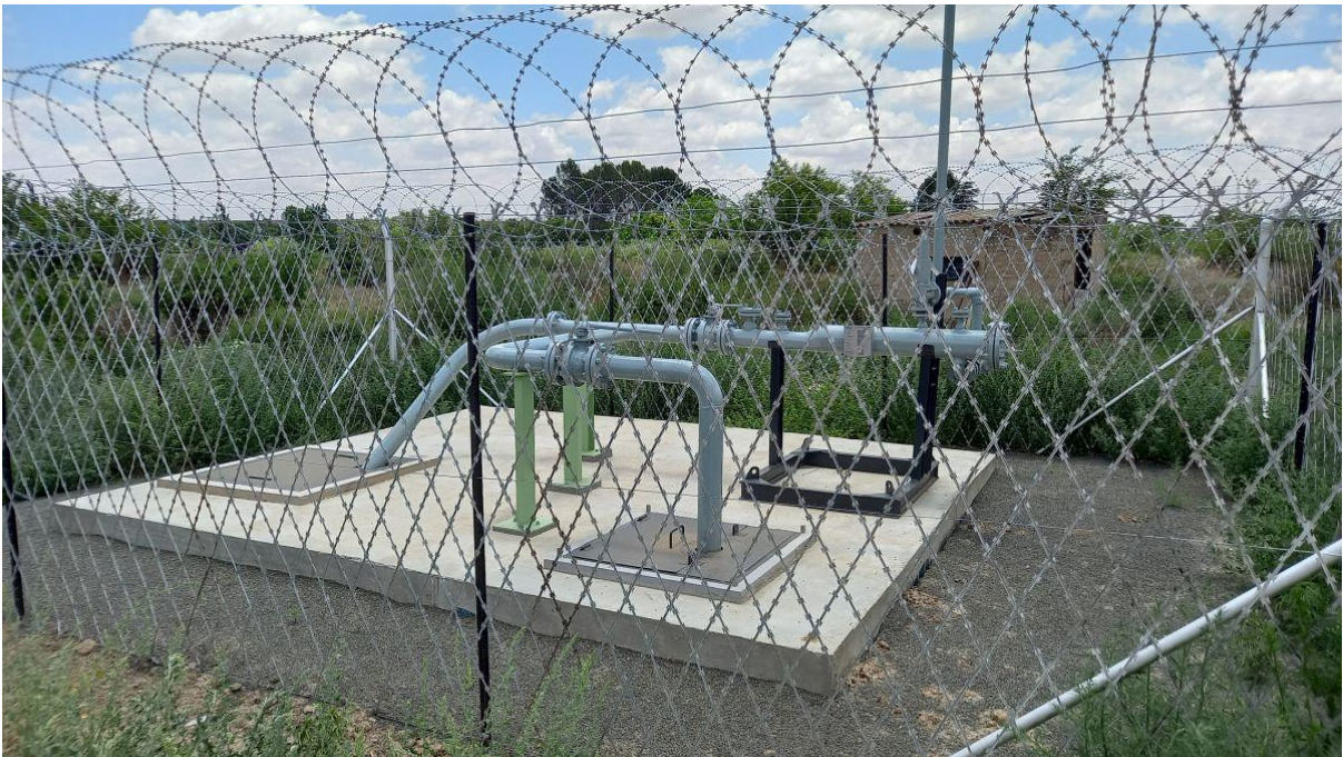
Figure 9: Construction work at the pigging stations were completed.
