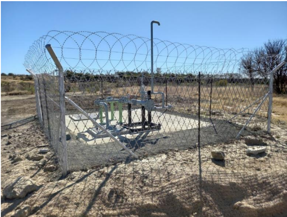
Figure 13: Installation of the pigging stations was completed.
