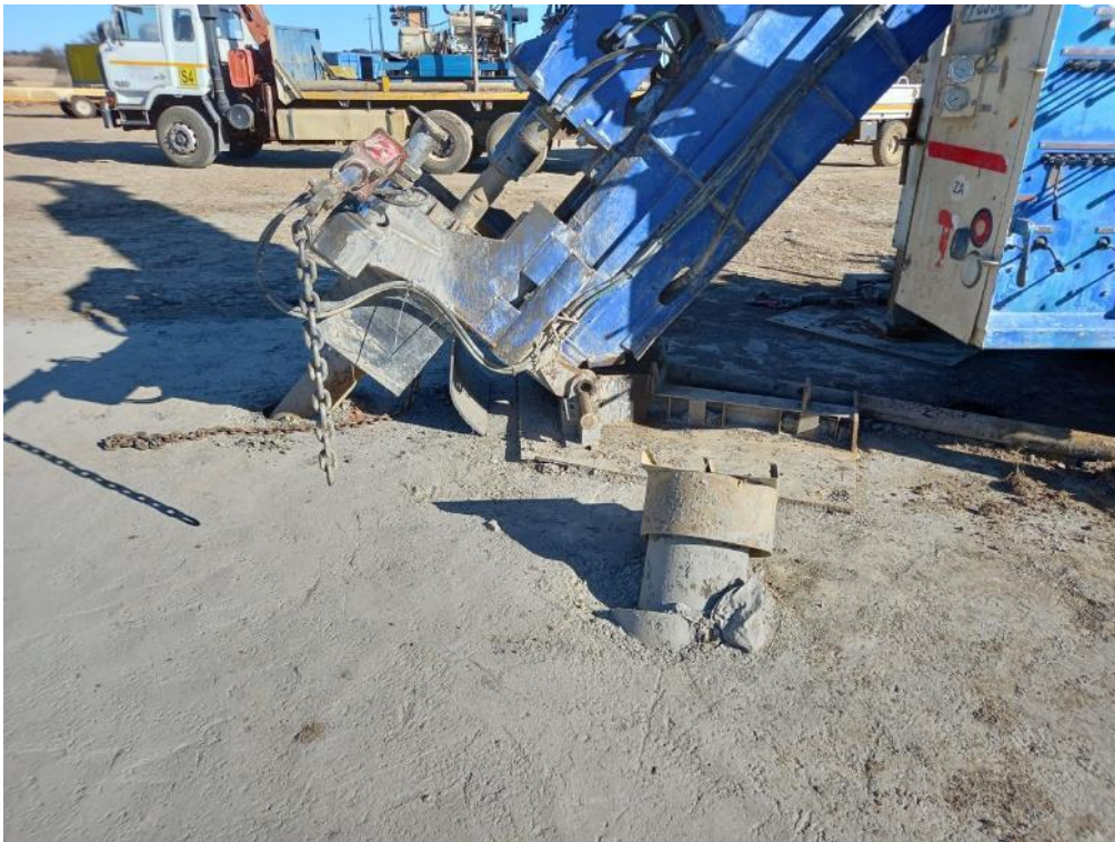
Figure 17: Installation of the casings at wells R2D2 and C3PO continued.
