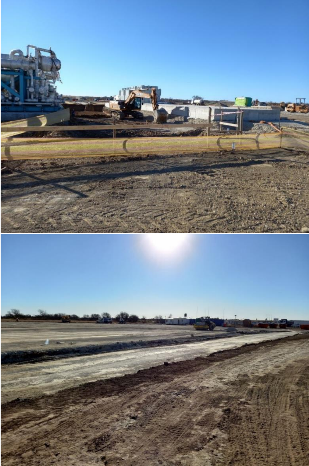
Figure 7: Layer works at the platforms of the LNG/Helium process plant complex.
