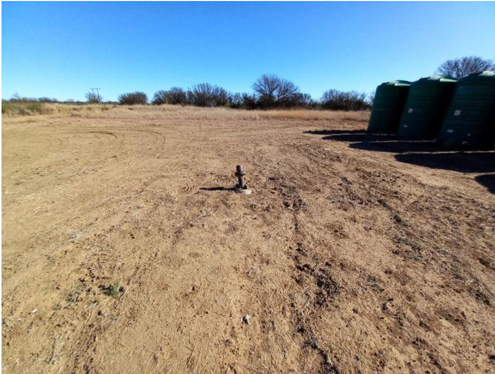
Figure 20: Rehabilitation around exploration well P2V2 was not completed.
