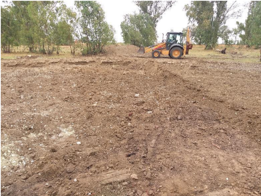
Figure 3: Topsoil stripping at the EX01 well site commenced.
