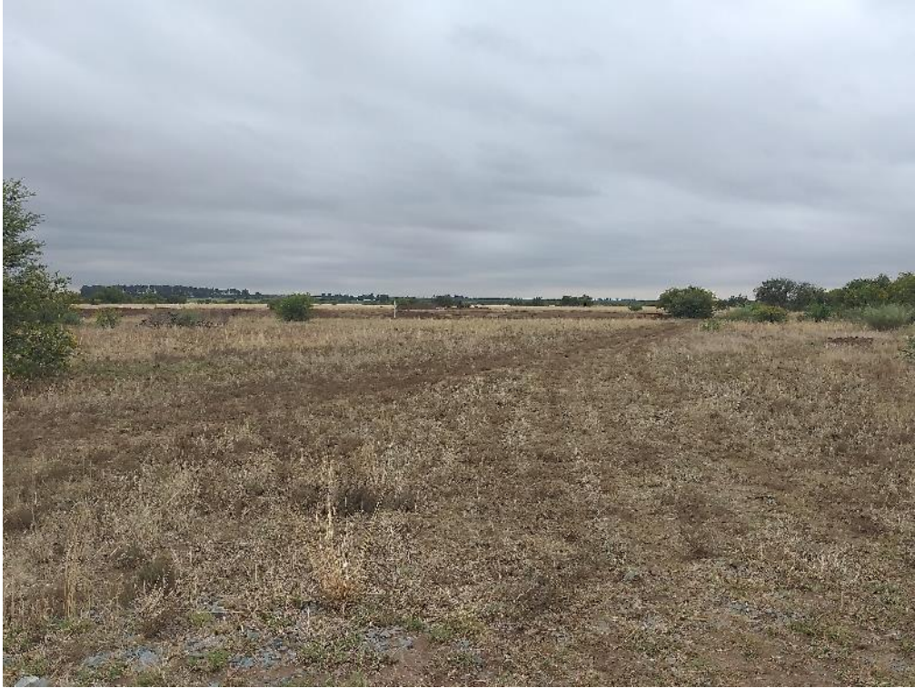
Figure 2: Topsoil stripping for the construction camp, near HDR1 commenced.
