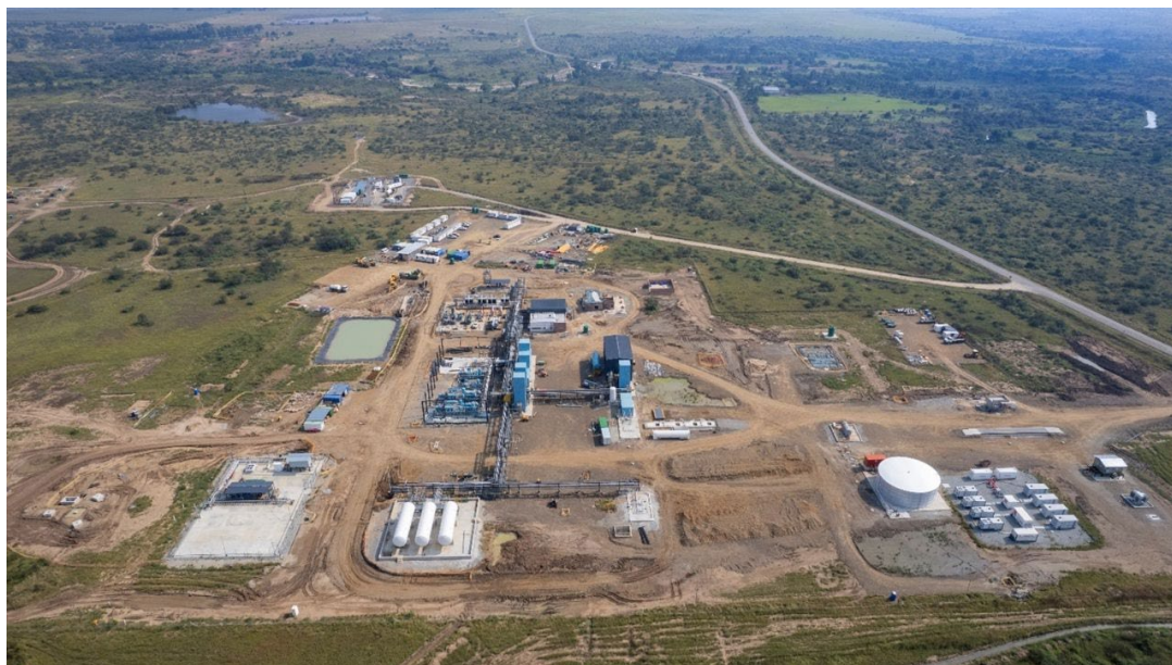
Exhibit 2 – Aerial shot of RLT's Virginia Gas Project, Phase 1
